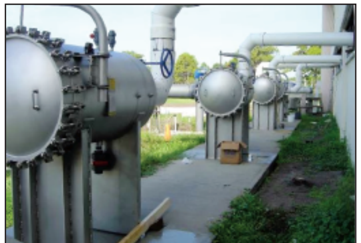
Figure 2. Temporary Cartridge Filter Header
