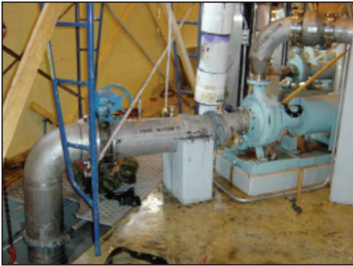
Figure 3. New Stainless Steel Feedwater Pump Header
