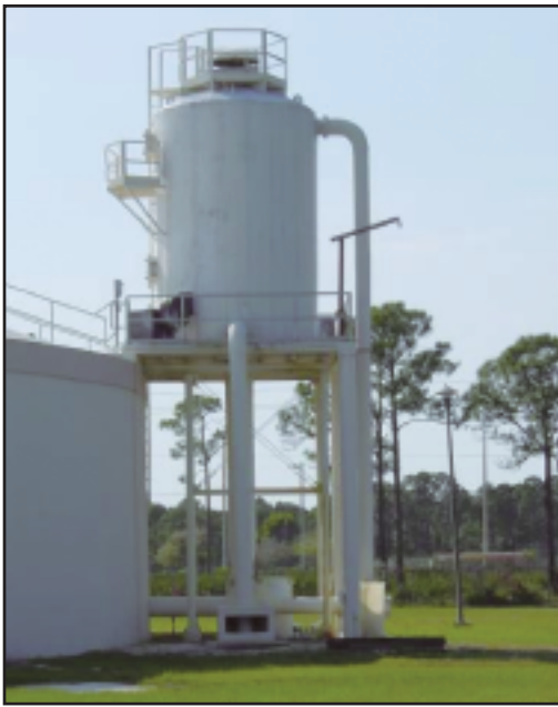
Figure 6. Existing Degasifier
