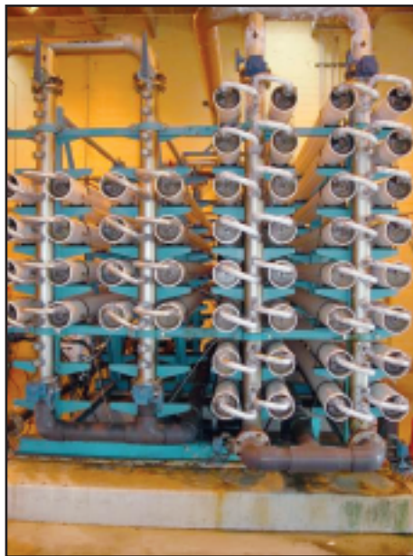
Figure 5. Typical RO Train Array
