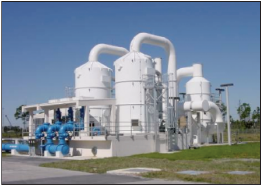
Figure 7. New Post-treatment System
