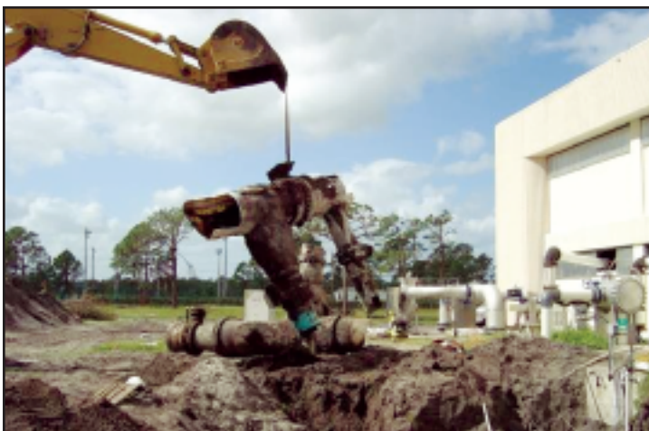
Figure 1. Removal of FRP Piping
