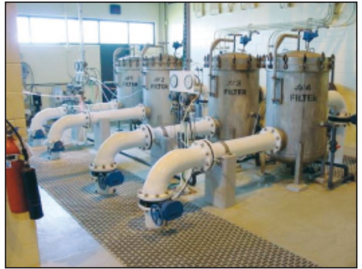
Figure 4. Old Filter Vessels
